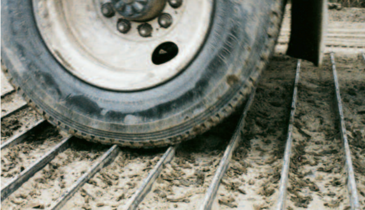
TYPICAL USE ON MATERIAL IMPORT/EXPORT JOB SITE
